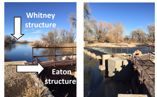
POI #1: Eaton ditch head gate with Whitney ditch diversion in background (looking upriver) and Eaton diversion structure with head gate (looking downriver)
