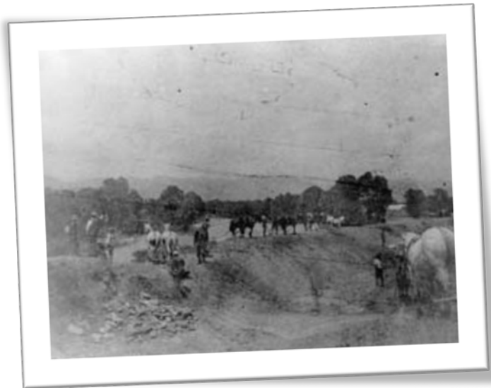
Early irrigation ditch construction in Fort Collins: photo courtesy of A.A. Edwards (early pioneer) c/o of history.poudrelibraries.org
