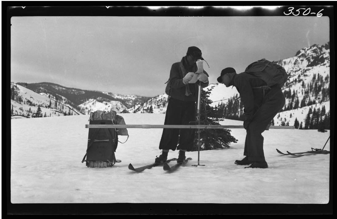
Figure 10. Measuring the snow pack in a Northern Colorado snow course. The person on the left is holding a cylinder of packed snow extracted from the snow pack. The person on the right is weighing it. Photo courtesy of Irrigation Research Papers, Water Resource Archive, Colorado State University.
