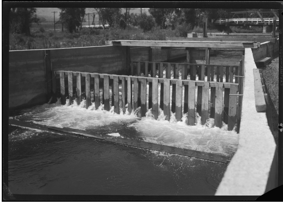
Figure 3. Water passing through riffle deflectors during an experiment at the Bellvue Hydraulics Lab. Photo courtesy of Irrigation Research Papers, Water Resource Archive, Colorado State University.
