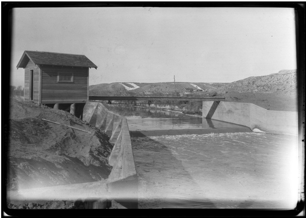
Figure 5. Forty foot Parshall Flume installed near Ft Lyon, Colorado, near the Arkansas River in 1932. Photo courtesy of Irrigation Research Papers, Water Resource Archive, Colorado State University.
